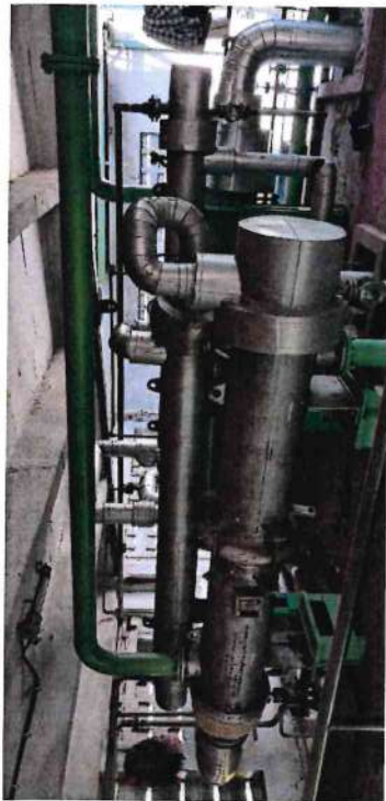
Photo -5 (Reflux Condenser)
